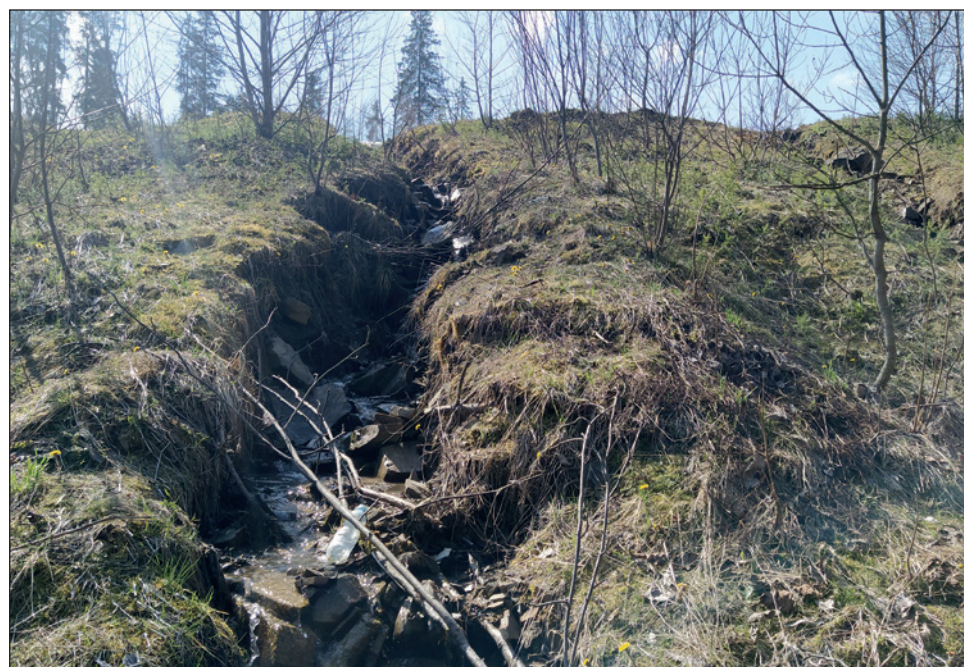
Fig. 10. Perpendicularly routed, newly deepened drainage ditch, Jaworzyna Krynicka
